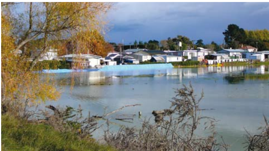
Waitaki Bridge settlement protected from flood waters by inflatable barriers
